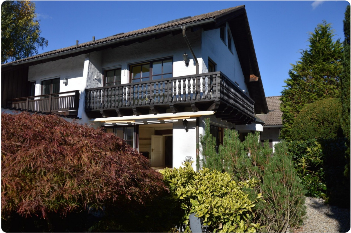
View of the house from the garden
