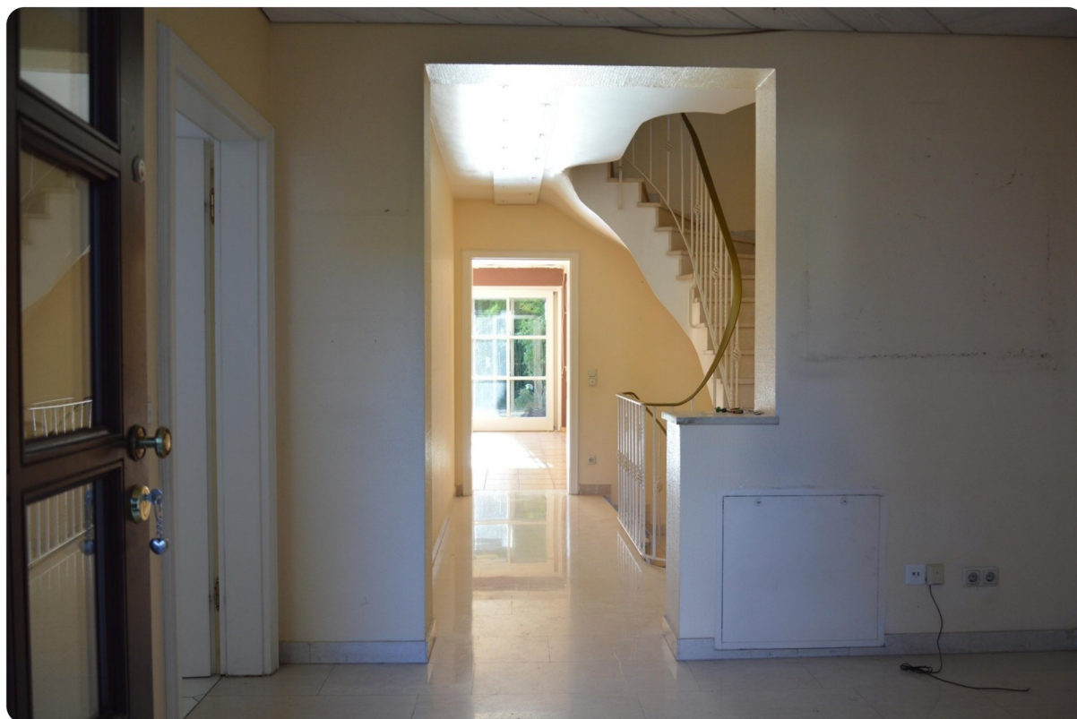
Ground floor hallway
